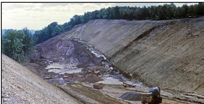
Figure 9. Excavation for a cutting along the re-aligned A38 (Exeter-Plymouth) road, after torrential rain created the gully in the cut slope to expose a complete section through the local sequence of the Upper Greensand.
